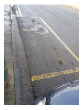
Figure 5.4: Accessible parking bay with no ramp
